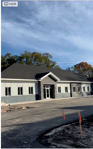
Construction Progress as of Dec 2023
